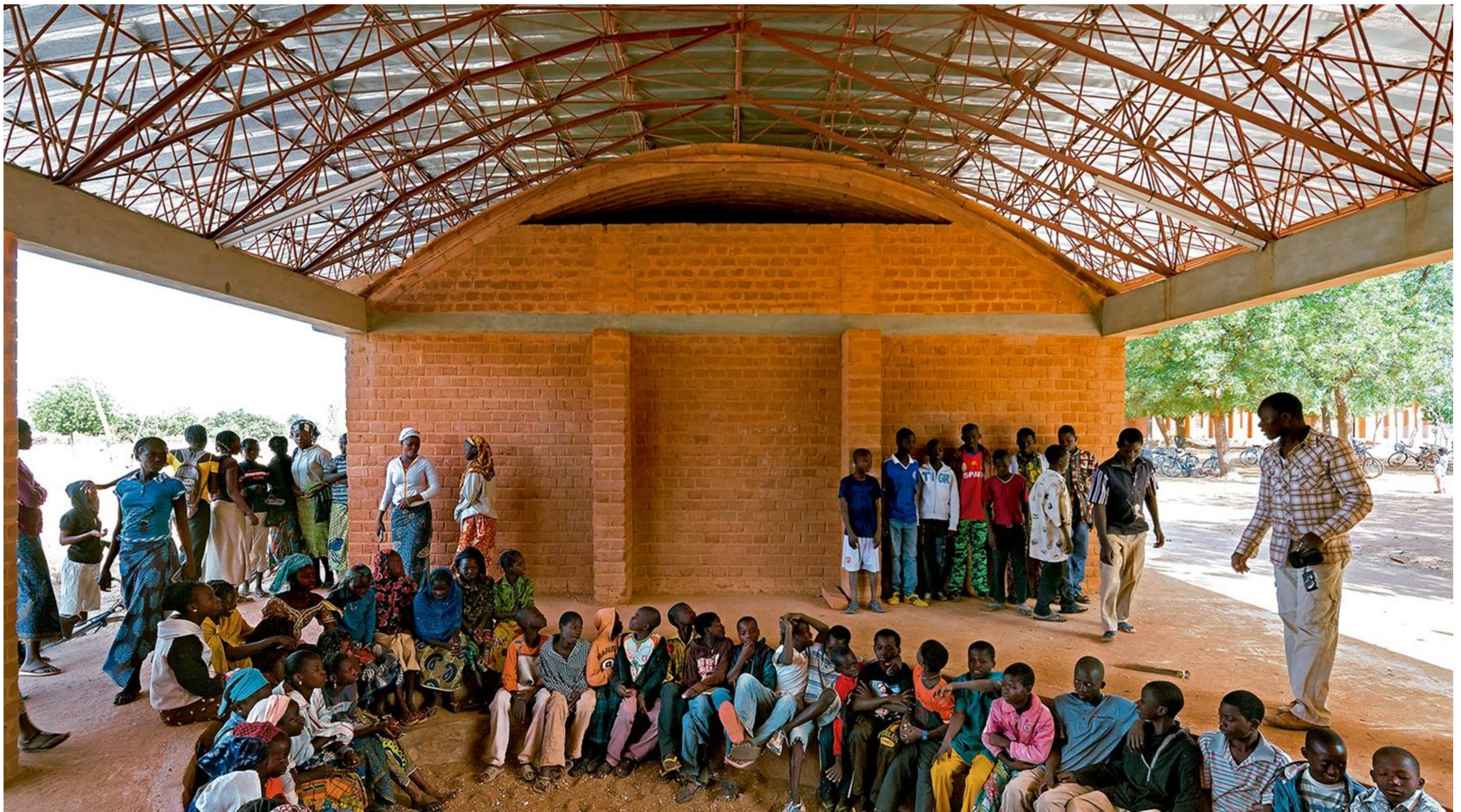
Primary school, Gando, Burkina Faso / Francis Kéré / 2003-2008
