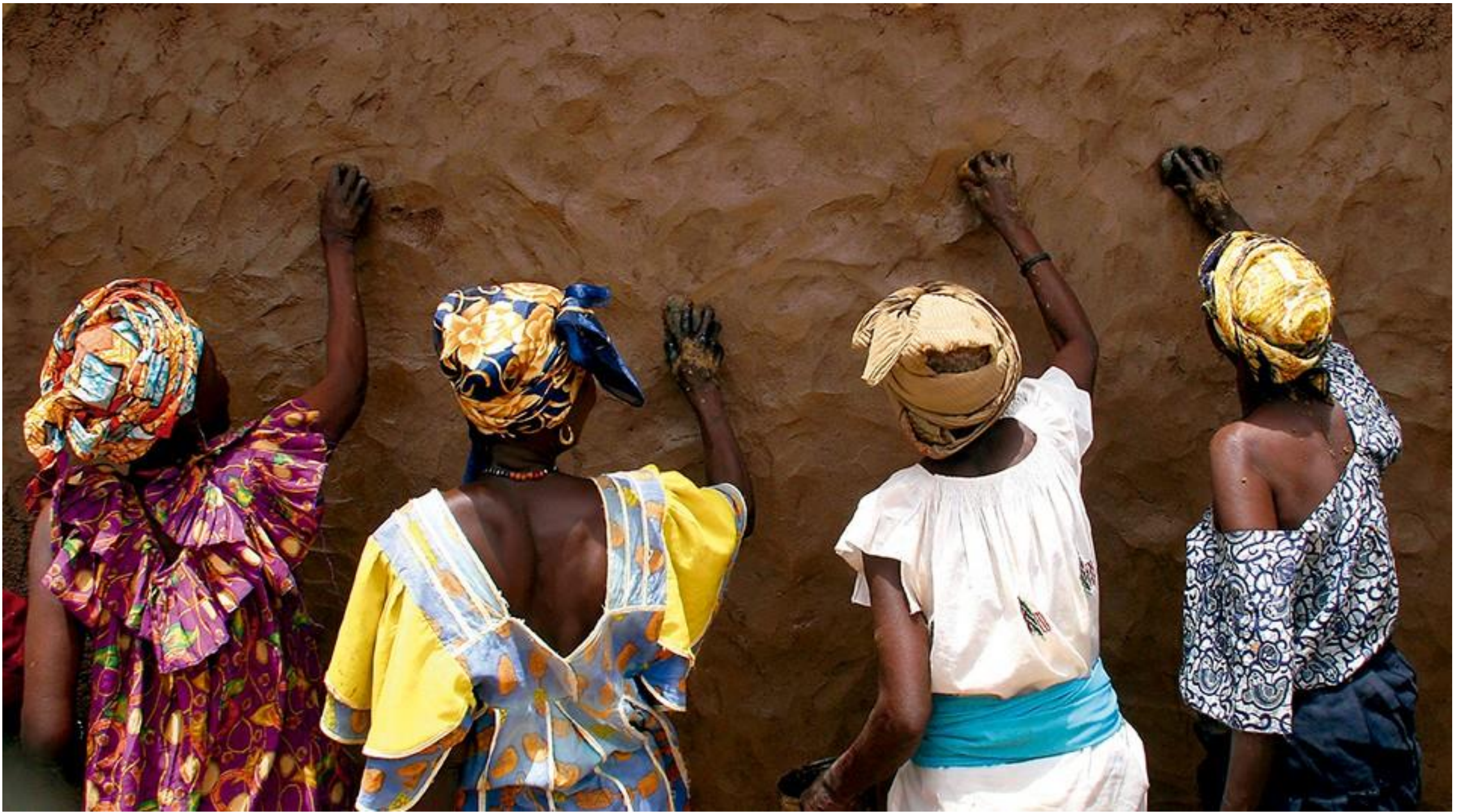
Primary school, Gando, Burkina Faso / Francis Kéré / 2003-2008
