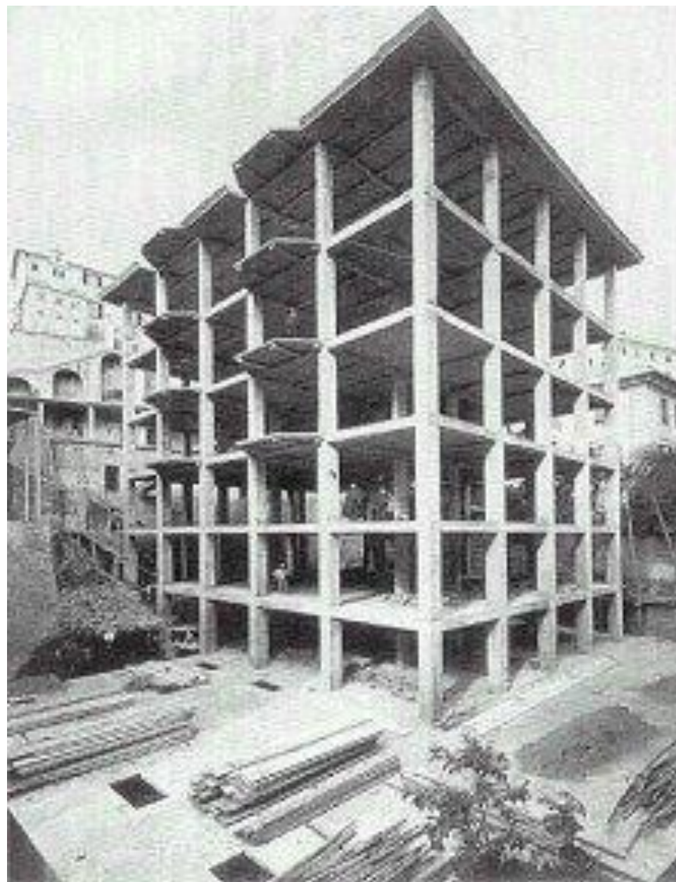
Fig. 12. System of reinforced concrete, by Hennebique (from Whittick, European Architecture 1).
